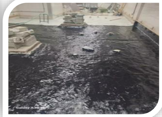
Pantry Area Waterproofing
