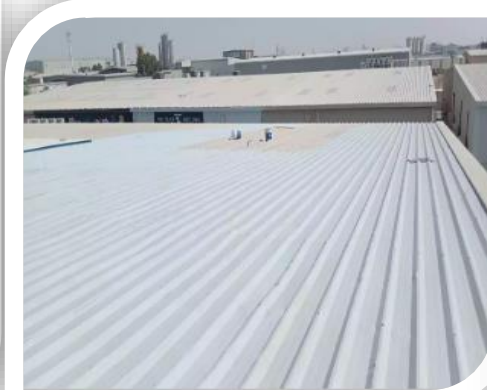
Metal Roof Waterproofing
