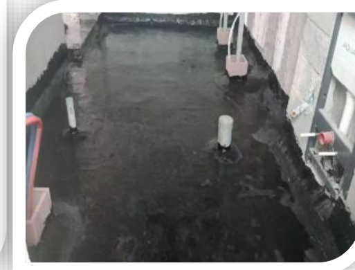
Bathroom Waterproofing
